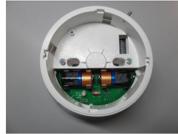
Picture 6 - primary and secondary batteries inserted
