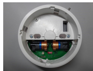
Picture 6 - primary and secondary batteries inserted
